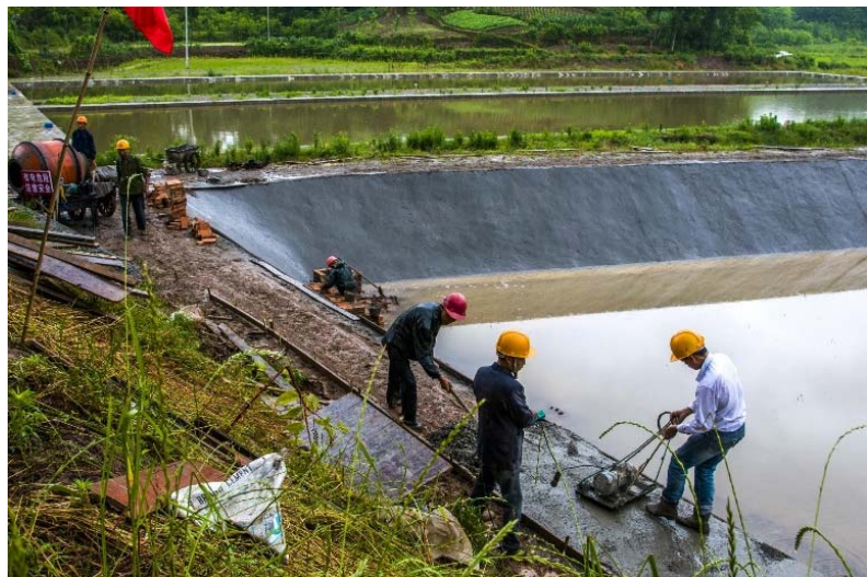
冒雨施工(摄于拔山镇五星村)
